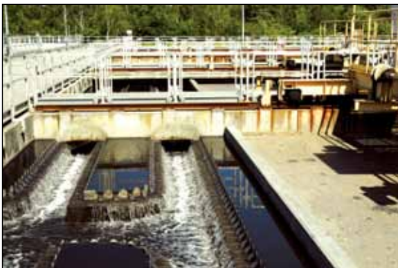
Monitoring Water Flow at a Wet Station
